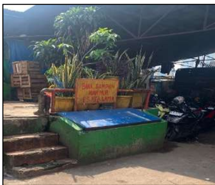
Figure 6. Condition of Kebayoran Lama Market Waste Bank, Area 11
